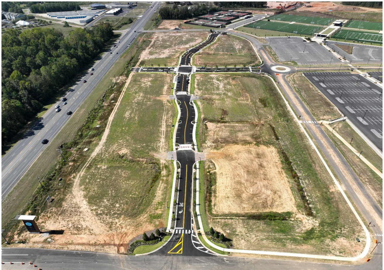
Aerial showing completed Marketplace infrastructure.
